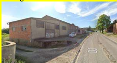
Ancienne station essence/garage
